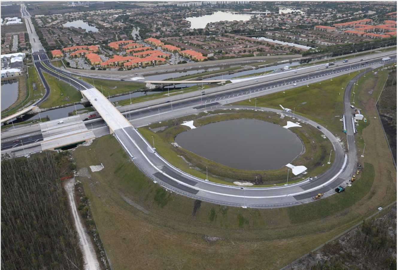
Florida's Turnpike / Northwest 74 th Street Interchange
